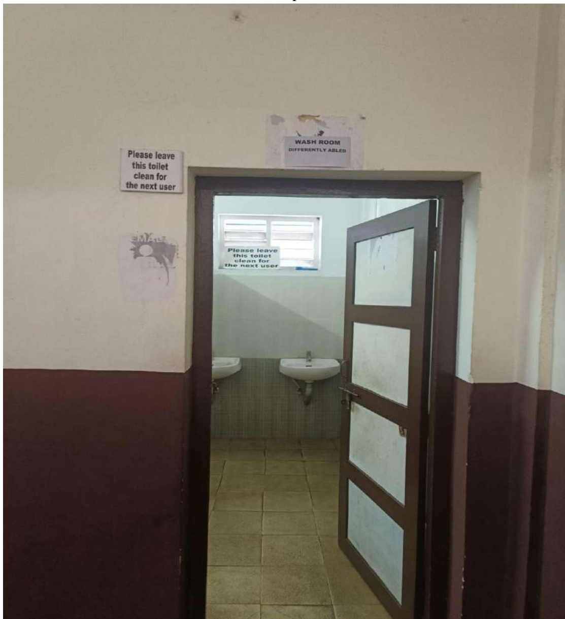
Washroom facility for differently abled
