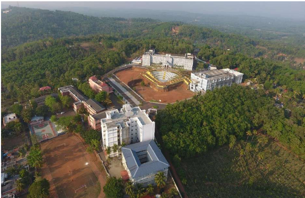
Mangalam College of Engineering- Campus
