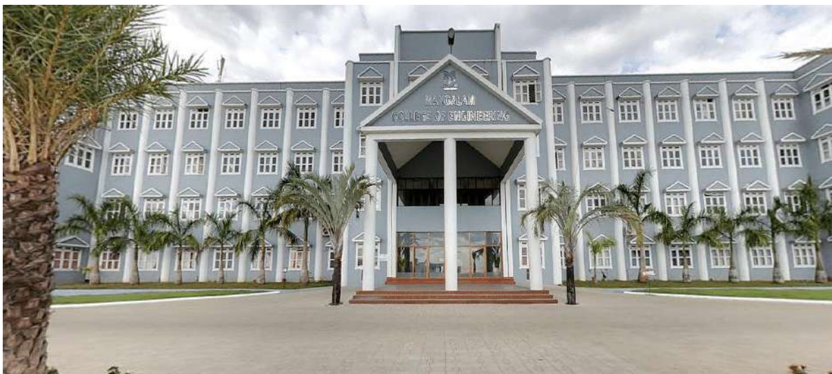
Mangalam College of Engineering- Campus
