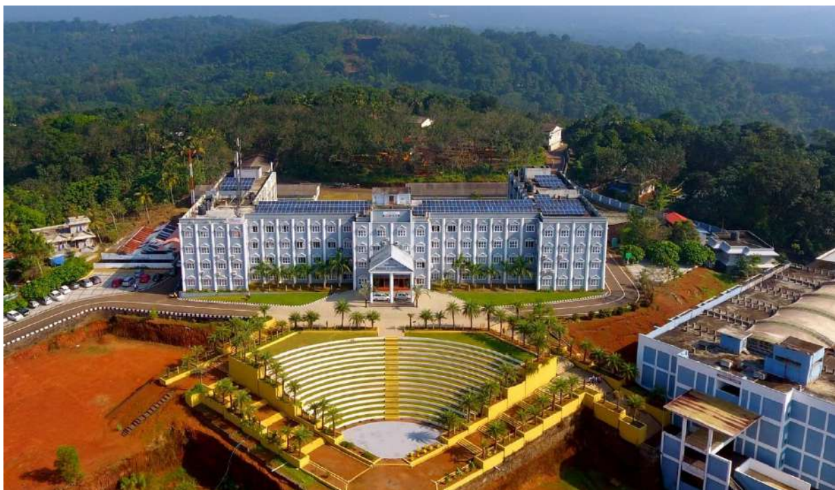
Mangalam College of Engineering- Campus
